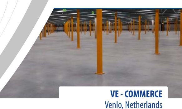
Warehouse - SFRC ground bearing Ultimate® 'seamless' floor slab
