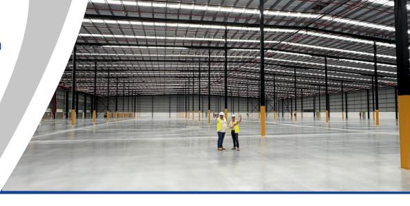
By supplying AFT+0960HE fibres at an optimised dosage of 23kg/m³, the project benefited from a steel fibre reinforced slab that achieved both performance and aesthetic goals. The fibres provided excellent crack control and enhanced load distribution — essential for a facility designed for high rack storage, heavy forklift traffic, and long-term durability.
