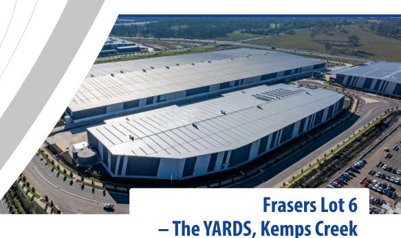
Twintec supplied AFT®+0960HE steel fibres for the Lot 6 – The Yards development by Frasers Property. Designed to handle heavy-duty industrial loading with 8-tonne post loads, the project required a robust reinforcement solution. At a dosage of 28kg/m³, our AFT®+0960HE fibres provided the strength, ductility, and crack control necessary for long-term slab performance.
