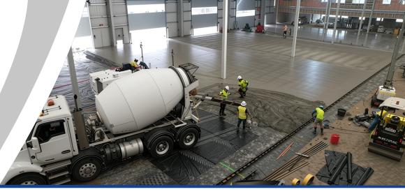
Beyond aesthetics, the AFT®+0960HE is designed to enhance the performance of modern industrial floors. Manufactured from cold-drawn wire and anchored with hooked ends, the fibre provides superior crack control, toughness, and ductility in concrete. By replacing or supplementing traditional reinforcement, it enables the construction of jointless and seamless slabs, external yards, and ground slabs on piles — delivering faster installation and reduced maintenance over the life of the floor.
